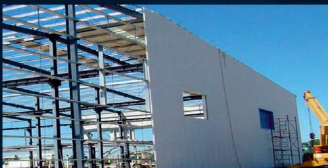
Roof & Wall Sheeting
