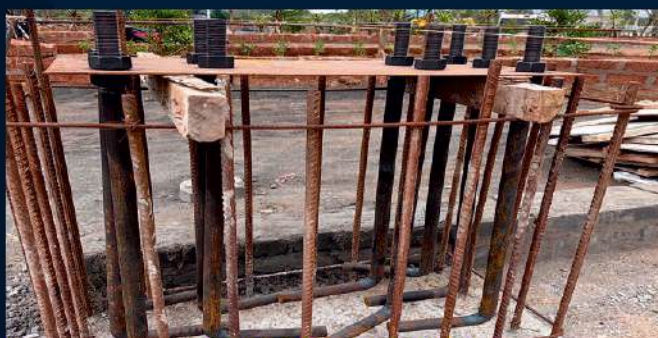
Anchor Bolt Mounting
